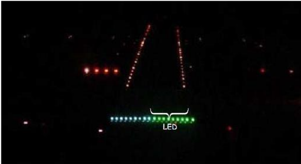
Figure 5- 10 LED and incandescent threshold lighting
